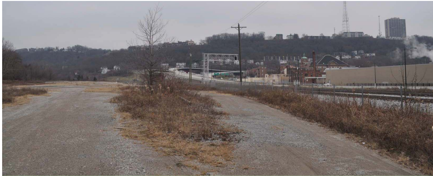
11 On site looking west
