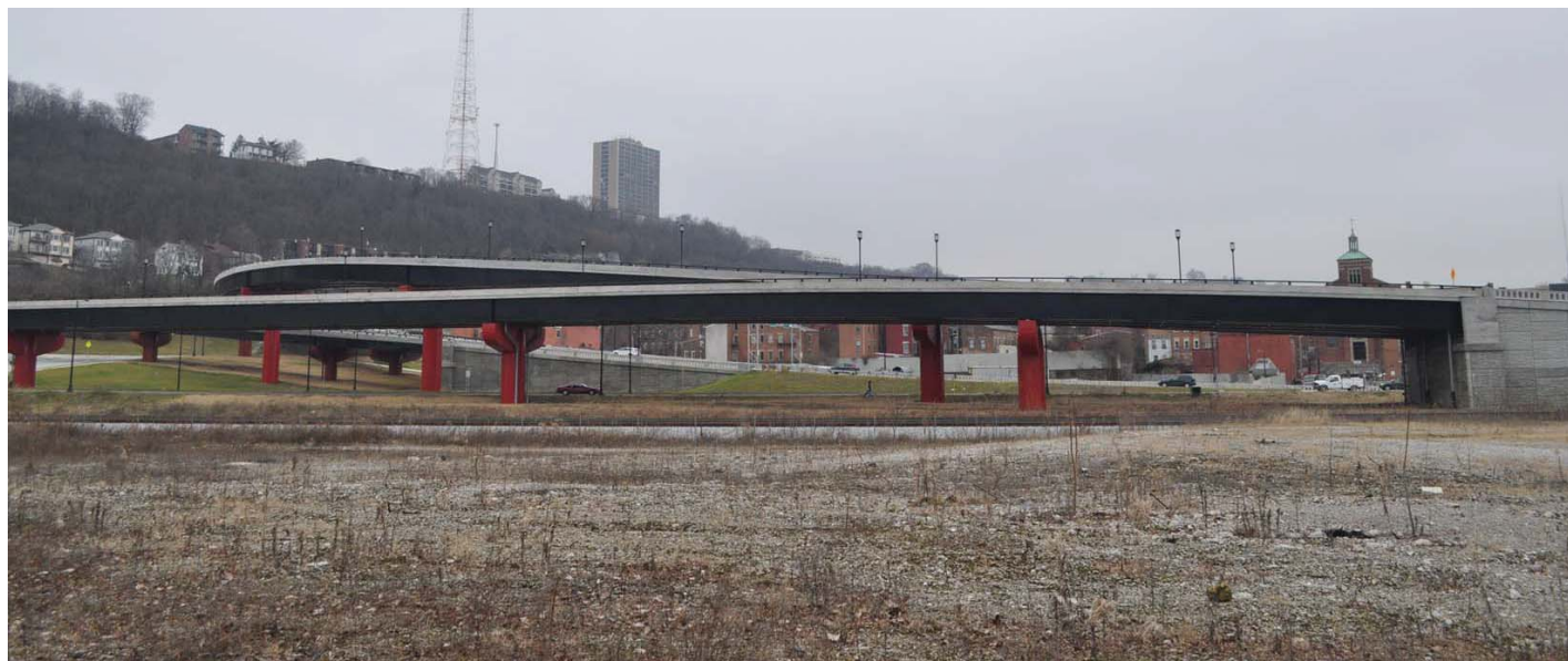
17 On site looking north toward Lower Price Hill
