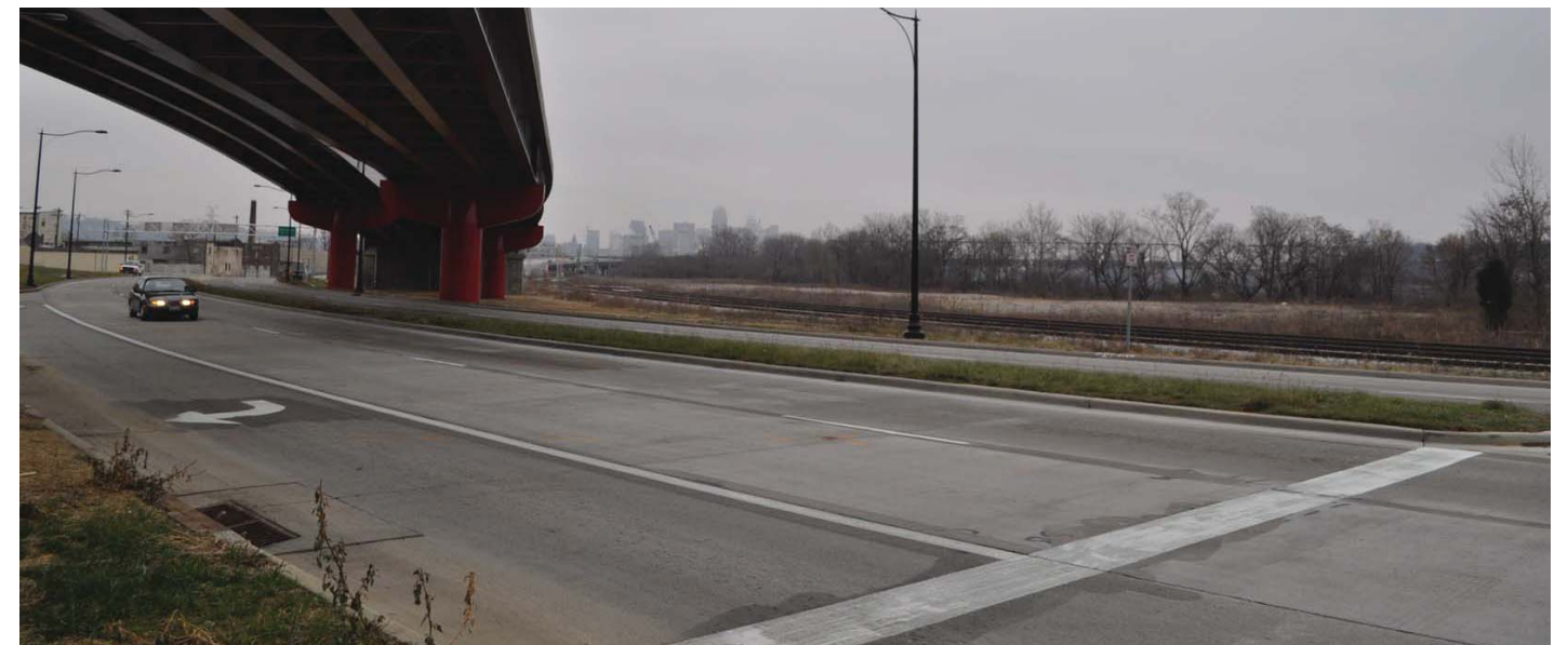
22 Looking southeast, at site, from State Avenue (#1 of 4 picture array)
